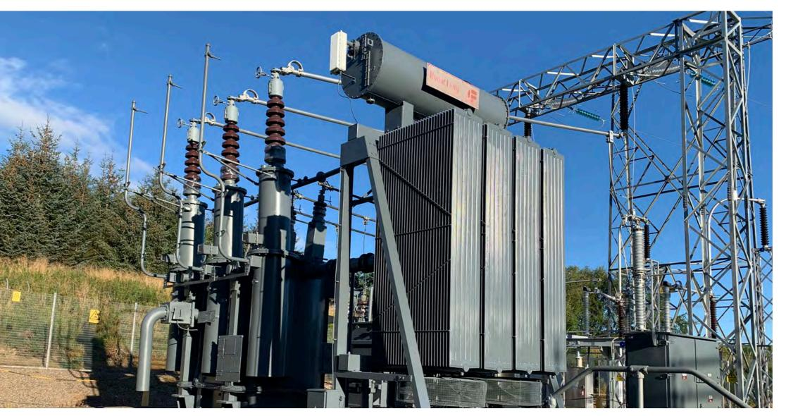
We recommend that transformers & auxiliary equipment are cleaned and painted every 5 years for coastal and marine environments and every 10 years for transformers located inland and within industrial environments. Transformers showing signs of corrosion can develop major issues such as tripping out of service or failure.
